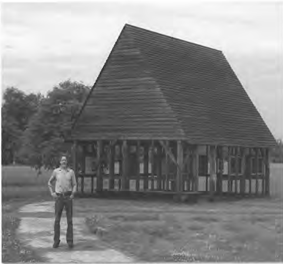
Peter Rivers and the Chapel Pavilion. Courtesy of Historic St. Mary's City.
